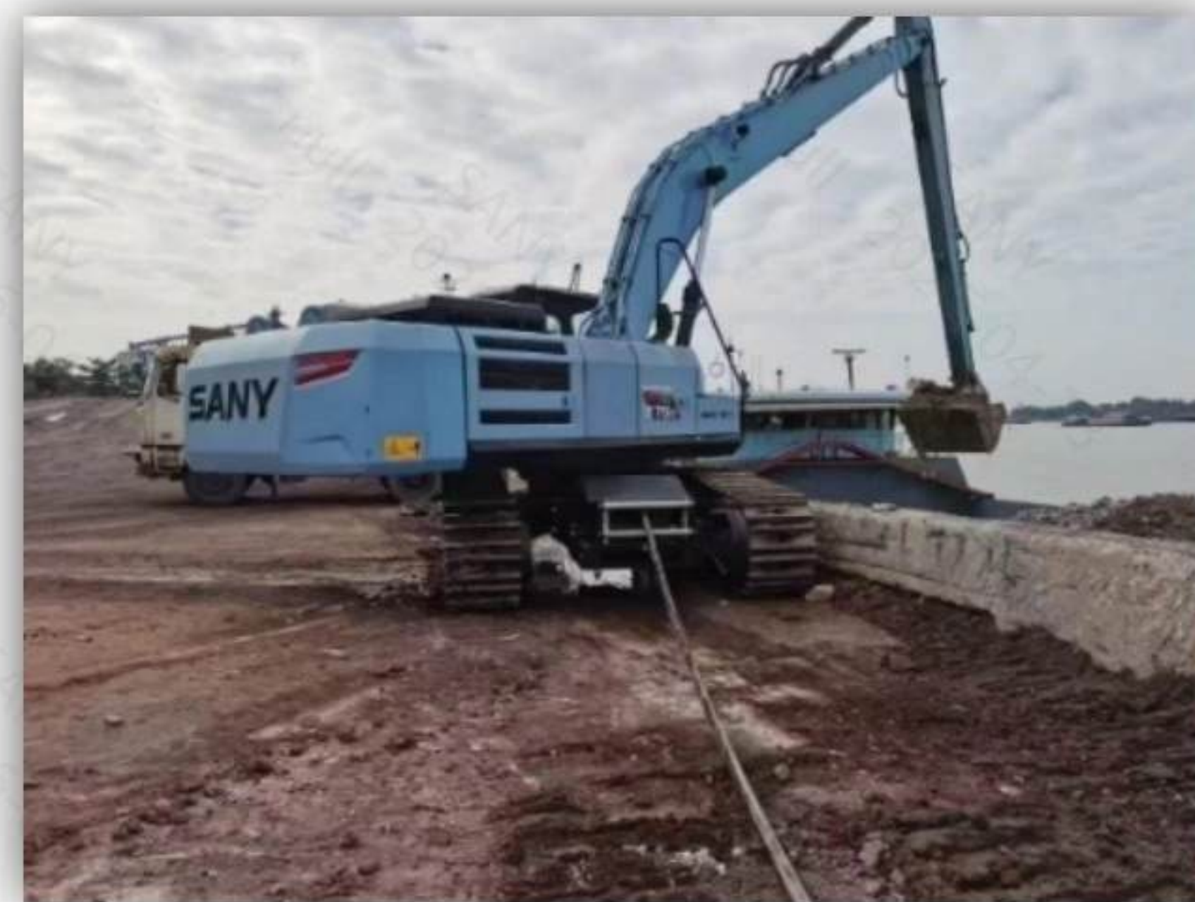
SY375E work in a dock with extended arm
