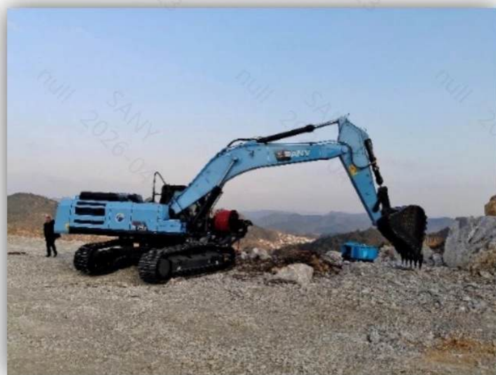
SY375E work in a rock mine with Electric roller
