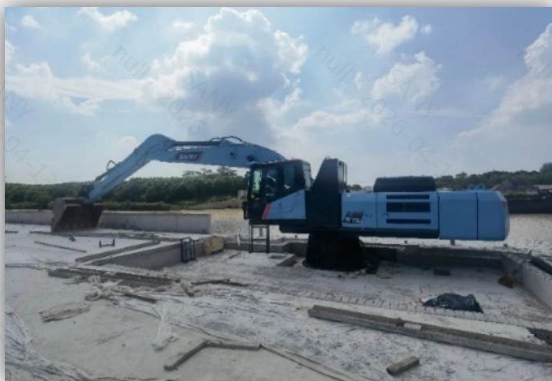
SY375E work in a dock with extended arm
